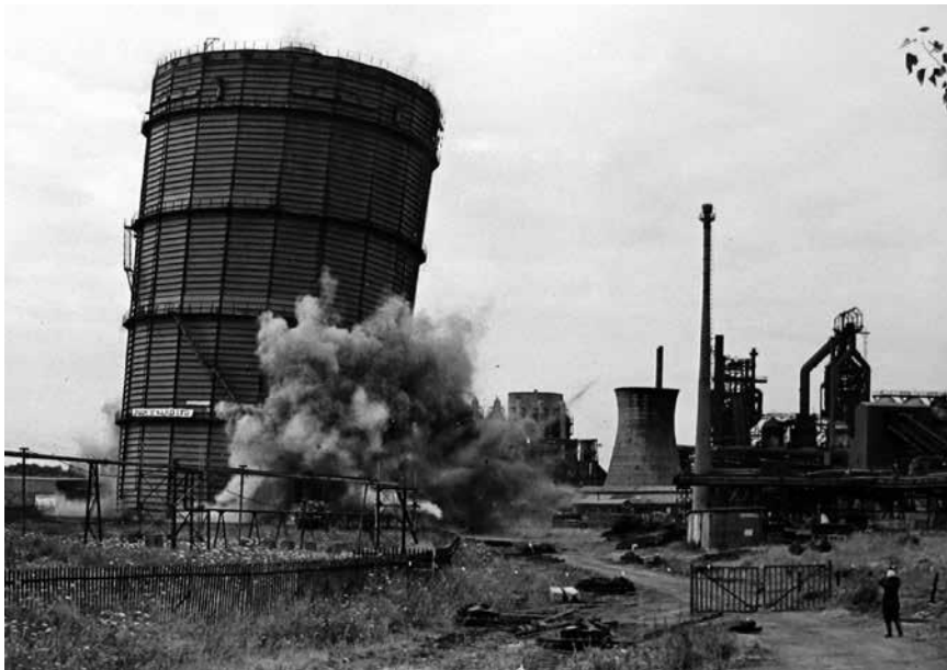
Demolition of the Steelworks
